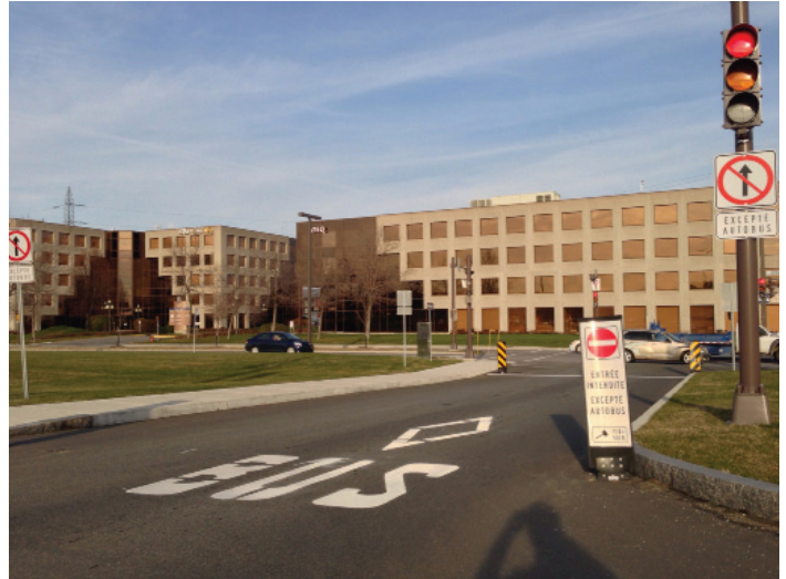
EXHIBIT 9: Example of Transit-Only Access to Transit Terminal in Quebec City
