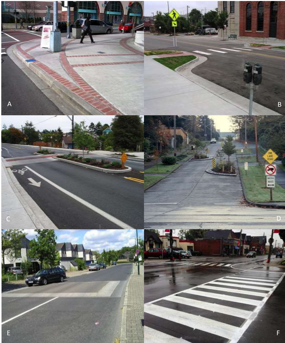
Figure 3.2: Common Traffic Calming Measures
