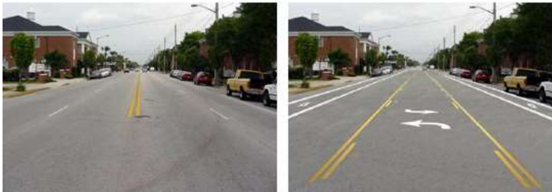
Figure 7.12: Edgewater Drive, Before & After treatment
