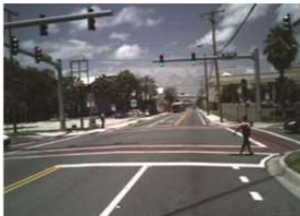
Traffic Signal Upgrades
