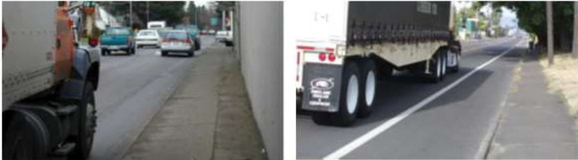
Figure 7.17: Before: Sidewalk dangerously close to traffic and, after redesign
